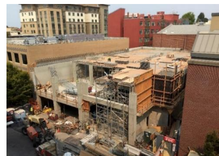
Progress on the 2009 Addison Street Workforce Housing project
